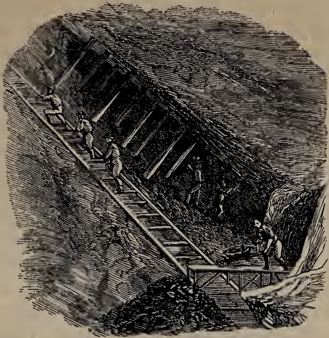
INTERIOR OF THE BODIE BUNKER.
